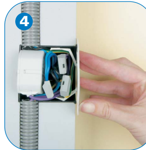
Incorporation of the actuator in the switch or installation box with cover
