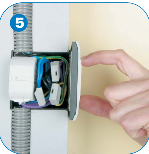
Installation of an actuator in the switch box with wireless push-button as a combined solution
