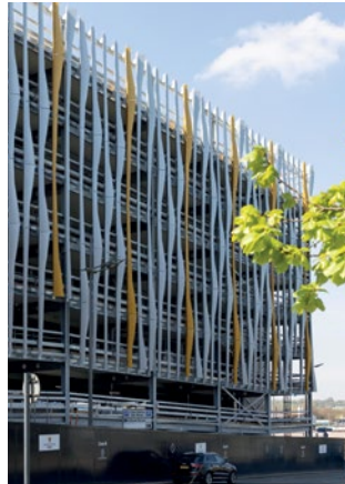
Multi-storey car park
