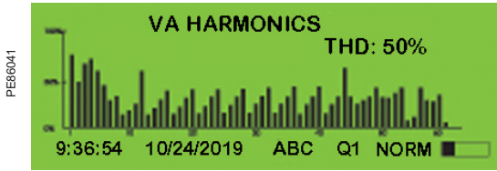
PowerLogic™ ION8650 front panel harmonic display
