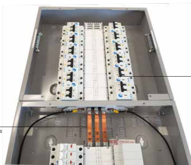
Busbar connection to existing boards
