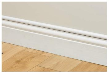
D-Line 20 x 10mm Micro+ profile gives a neat solution for single cables, while offering additional internal capacity that can be useful around corners.
