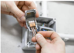
Place the wired connector in the Gelbox.
