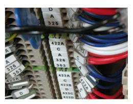
Part-used sheets are easily accomodated to avoid wastage. MG-CPM terminal block markers are available in versions to suit the particular clip formats of the most widely used products.
