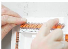
Snap the marking strips into the holder.
