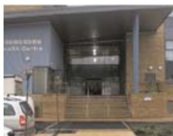
Todmorden House (Health Centre) Yorkshire
