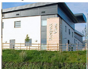
Prospect View (Health Centre) Worcestershire
