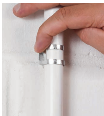
Secure conduit with locking tab
