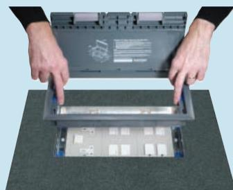
(1) The aperture dimension 203 mm has a fixing tolerance between 203 to 205 mm
