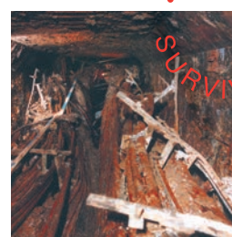
Pyro MI survived in this power station fire
