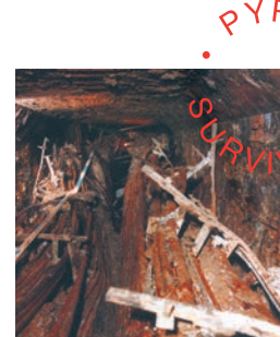
Pyro MI survived in this power station fire
