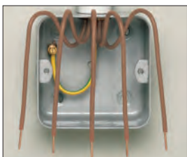
1 Install box and enter cables.
