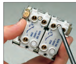
3 Fix switches into grid.
