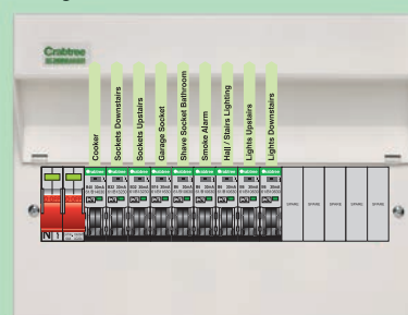
TT SYSTEM All independent circuits & 100mA Time Delay RCD
