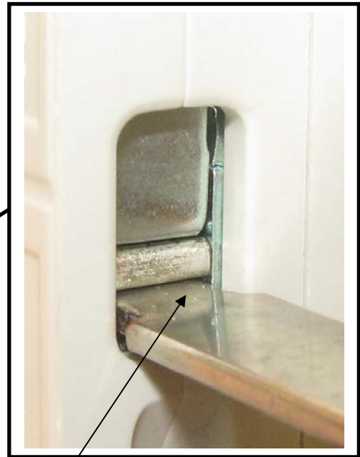
Busbar connection into lower cage, ensure cage is fully lowered before attaching to busbar
