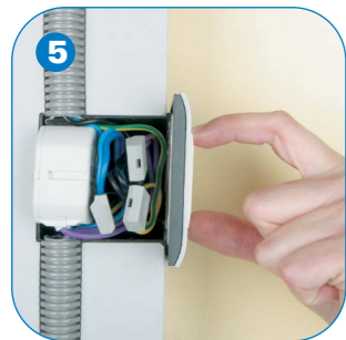
5 Installation of an actuator in the switch box with wireless push-button as a combined solution
