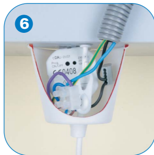
6 Installation of the actuator in the light fixture
