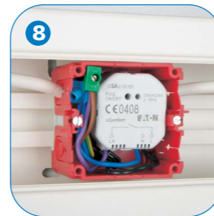
8 Installation of the actuator in a cable channel box
