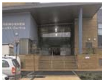
Todmorden House (Health Centre) Yorkshire
