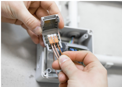
Place the wired connector in the Gelbox.
