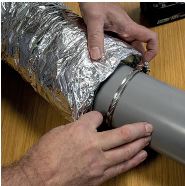
If fixing insulated or acoustic duct, pull the insulation fully over the connection.
