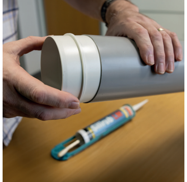
Carefully push fitting into duct
