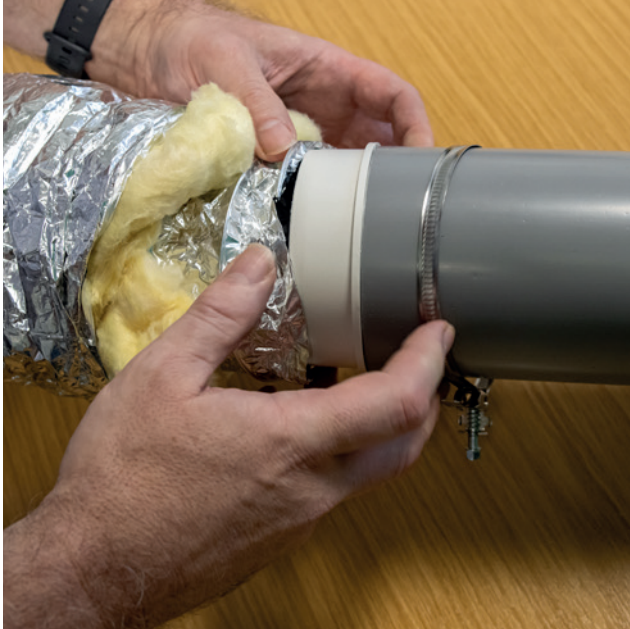
Carefully slide the flexible duct or inner sleeve over the connector
