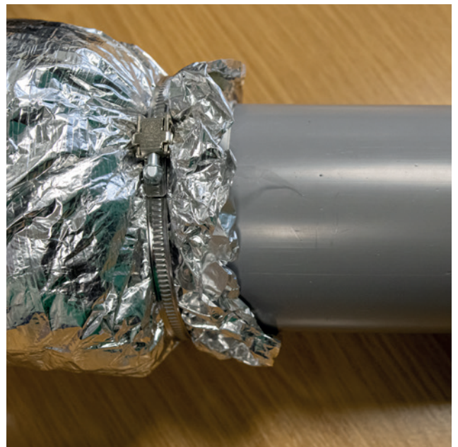
Pull the outer sleeve fully over the insulation and inner sleeve. Connect using a mechanical fixing and then tape (Do not use tape only)
