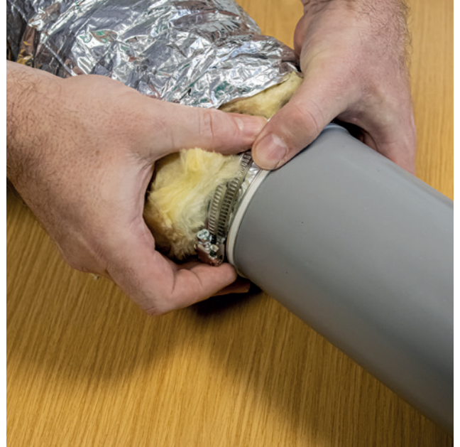
Apply a mechanical fixing (worm drive clip or strong tie wrap)
