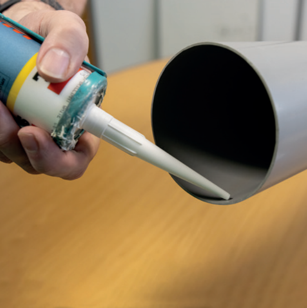
Apply a smooth layer of non hardening sealant/acrylic around the inside edge
