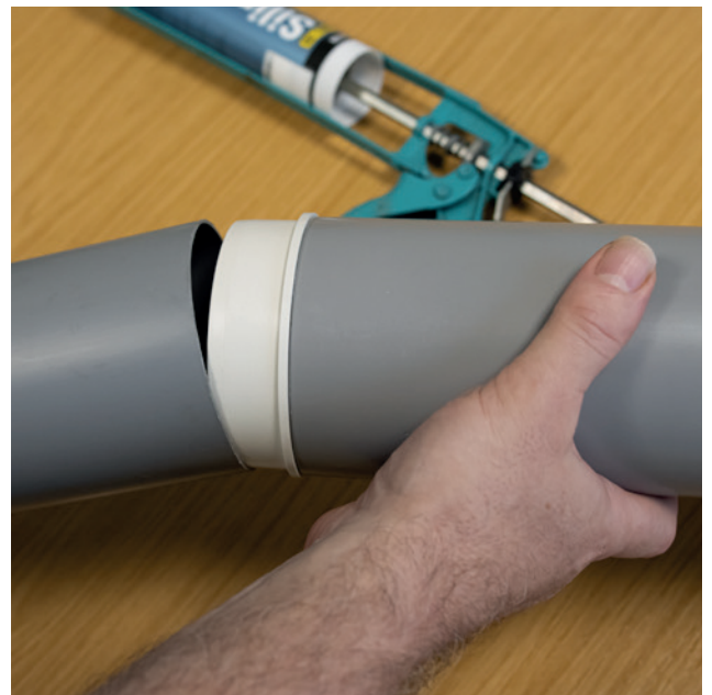
Carefully push the ducting onto the fitting
